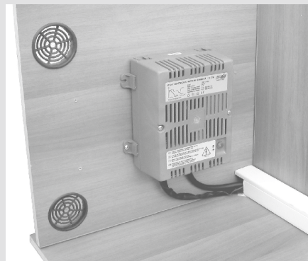
Fig.2 - INSTALLATION VERTICALE
